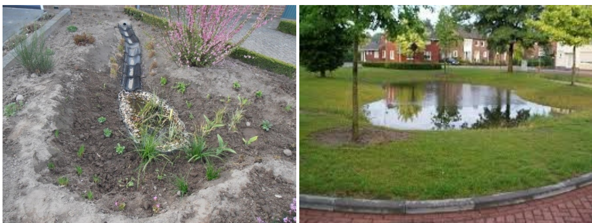
Figure 14: Rooftop runoff infiltration system (left) and a collective water retention and infiltration facility (right).
