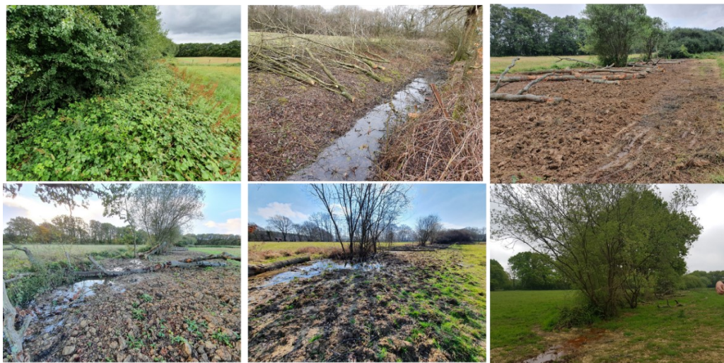
Figure 7 – Sub-site Harp Meadow. This sub-site included an agricultural ditch in a grassland. This was restored to a seasonal wetland in a similar way, filling in 100m of channel to restore a wet grassland.
