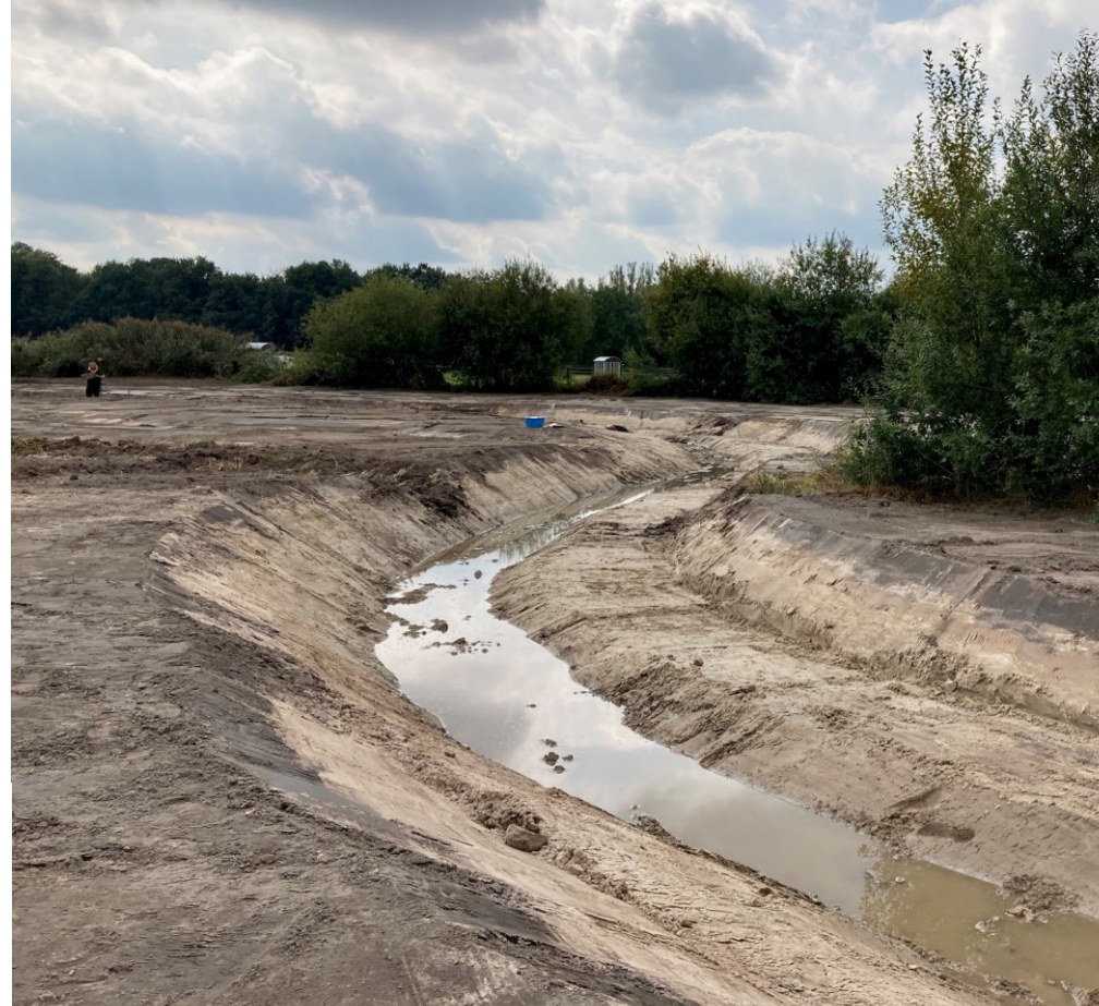
Restoration works in the Vloeiweide. A meander in the previously normalised brook Bijloop will be restored. Works are expected to be completed in Fall 2022.
